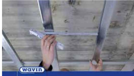
The panels are fitted with hooks that make fixing to the suspended ceiling structure possible.
