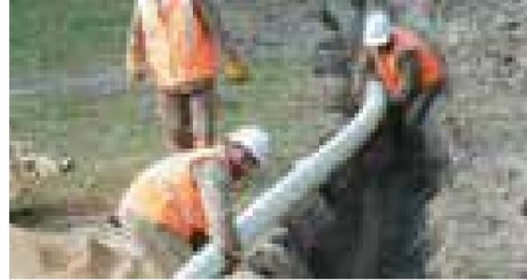
Apollo Plastic Pipes should be installed near the trench and then carefully laid at the bottom of the trench with the help of the installer inside the trench as shown in the below pictures.
