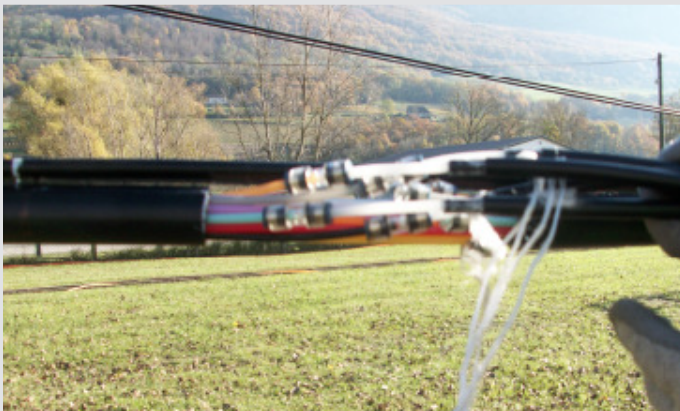
3. Connect the drop ducts on the connector and fasten the yarn to the Novonet Aerial using a tie wrap.
