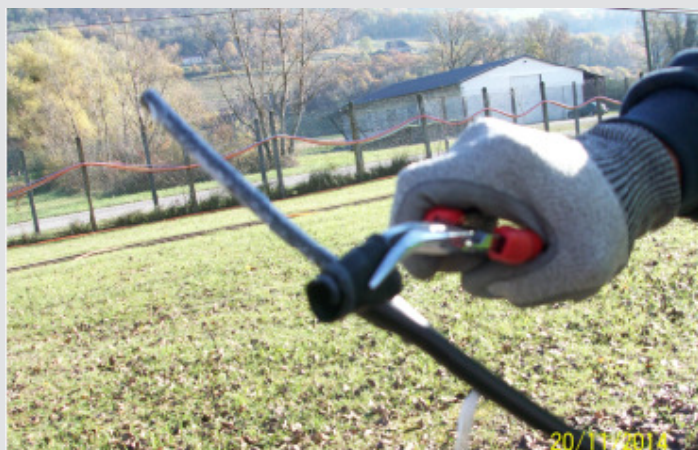
3. Remove the outersheath, using a standard pincer
