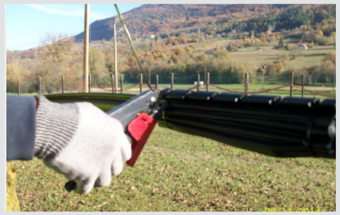
6. Tighten the gelwrap with cable ties using a tool.
