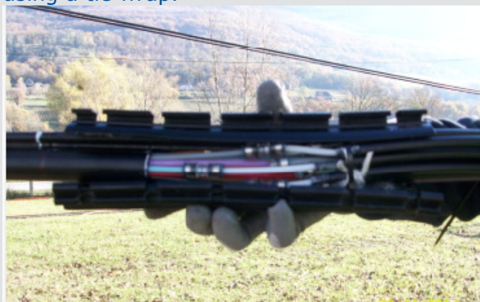
5. Place the gelwrap over the branch off and close it by firmly pressing the bottom part together.
