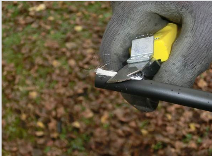
1. Remove the outer sheath of the drop at the place of the yarn with a cutter
