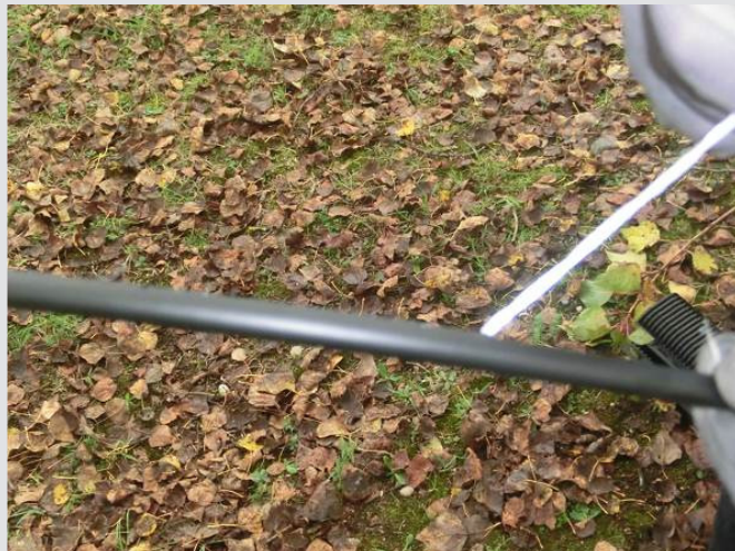
2. Cut the outersheath at a length of 20 cm with a microduct cutter and open it using the yarn as a ripcord.
