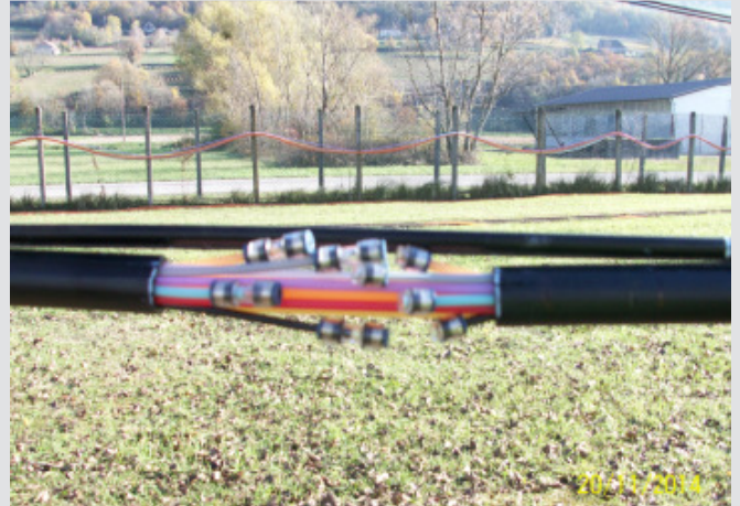
4. Connect the ducts with the connector, close the end with a endstop
