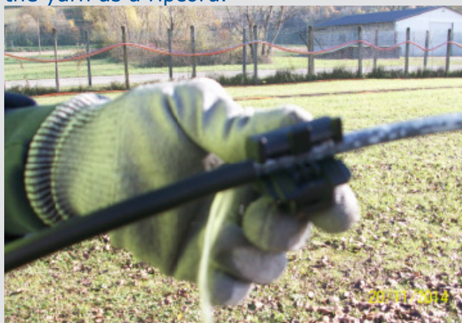
4. Cut the innersheath with the microduct cutter and remove it
