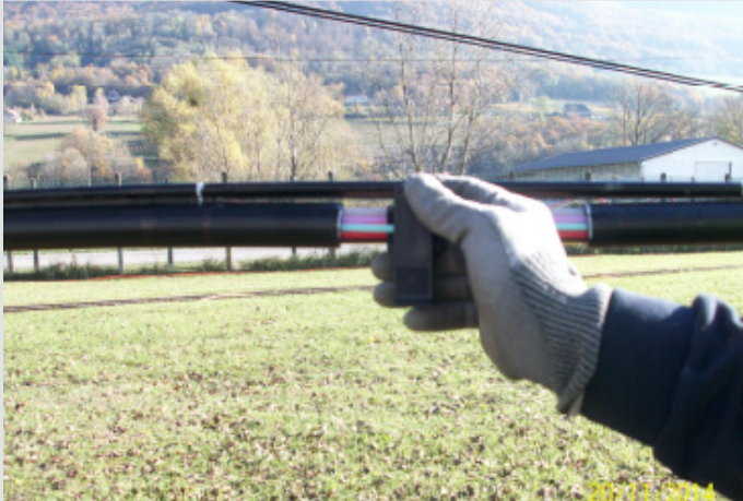
1. Cut the Microduct of the Figure 8 Novonet
