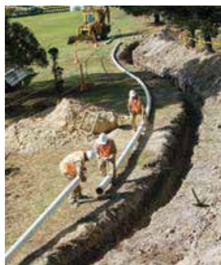
Connecting of the pipes can be done near the hood. The pipes are needed to be moved down with the help of an equipment in bearing line.
