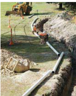
Connecting of the pipes can be done near the hood. The pipes are needed to be moved down with the help of an equipment in bearing line.
