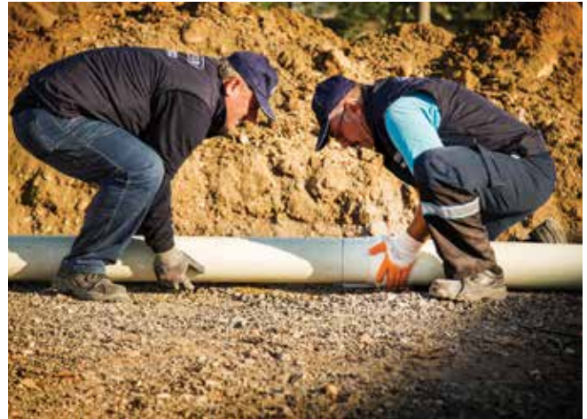
Push the pipe till the end of the mark of the pipe and use lubricant before the process.
