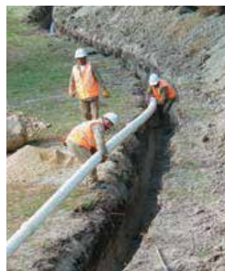
After putting the pipe into the trench by high care, sand or other filling material suitable with standards can be used.
