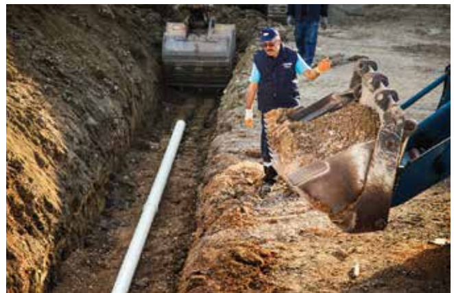
After putting the pipe into the trench by high care, sand or other filling material suitable with standards can be used.
