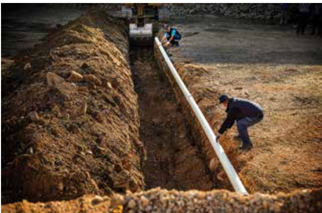
Connecting of the pipes can be done near the hood. The pipes are needed to be moved down with the help of an equipment in bearing line.
