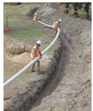
After putting the pipe into the trench by high care, sand or other filling material suitable with standards can be used.
