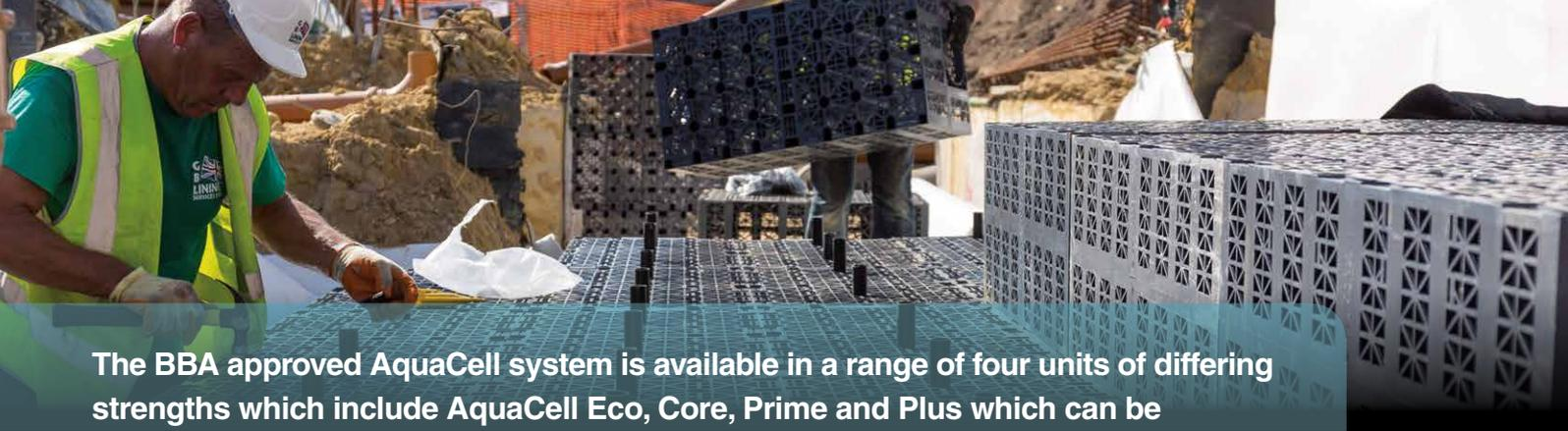
The BBA approved AquaCell system is available in a range of four units of differing strengths which include AquaCell Eco, Core, Prime and Plus which can be mixed and matched to create the optimum installation for a range of applications including landscaped or trafficked for either shallow or deep applications.
